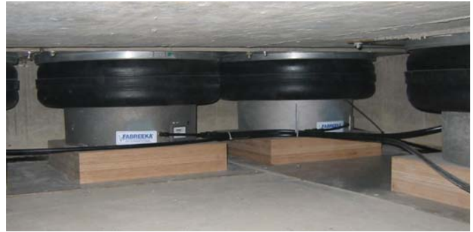
Air bag isolators provide a low natural frequency and large dynamic stroke where dynamic deflection is acceptable.
